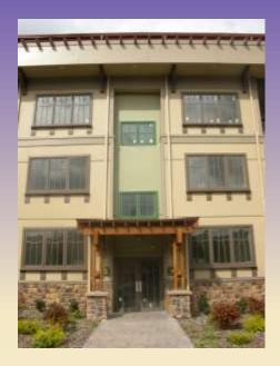
The privacy of each of the units front and rear patios is accomplished through both the building pod offset or/or stair towers. The four to ten-foot soaring roof overhangs gives the structure a sense that its floating like the lake.
